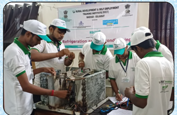
Action Photo of Refrigeration and Air Conditioning
